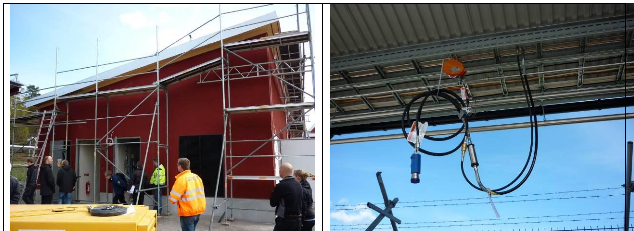
Figure 10. Left: Inspection of building with gas storage and electronic equipment. Right: The hose for slow filling is connected to the pipeline for the biogas which is placed in the roof.
