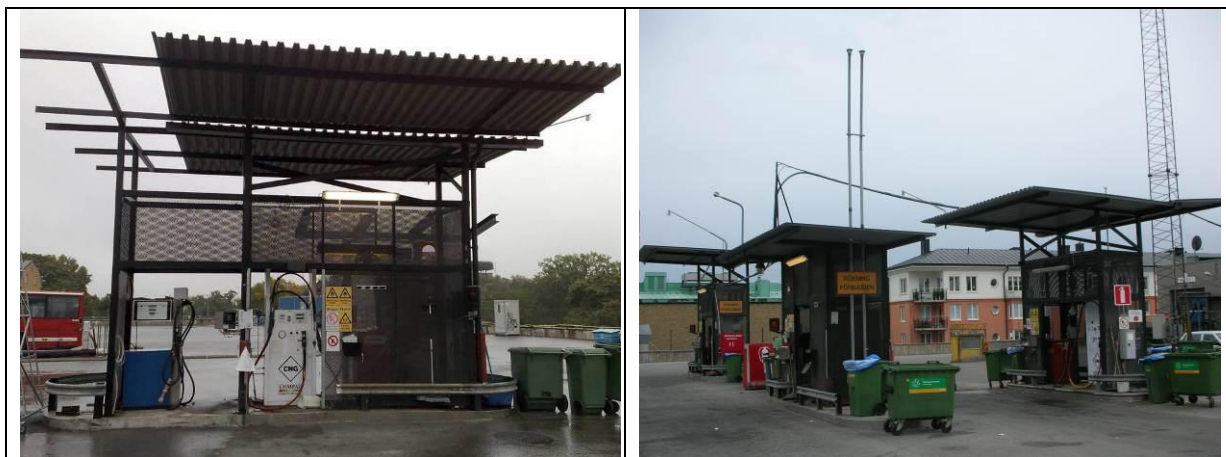
Figure 8. Fast filling dispenser for biogas and ethanol at SL's biogas bus depot Söderhallen.
